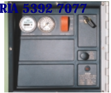
Curbside Instrument Panel Featuring SSAM, Shutdown System & Annunciation Module.
